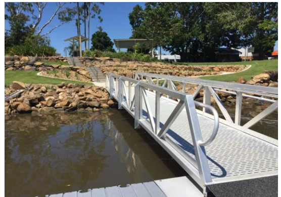
Figure 3 Pontoon and gangway installation, as well as disability access ramp to the gangway, at Budd Park, Murwillumbah, along the Tweed River.
