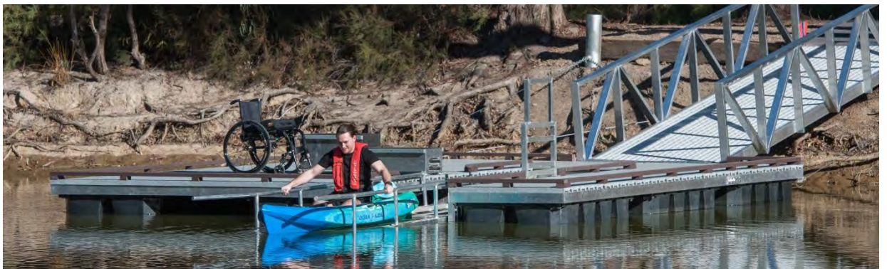
Figure 2 All-abilities access pontoon and gangway to support non-powered vessel use along Edward River.
