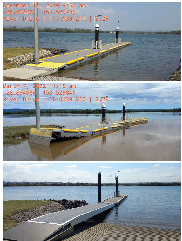
Figure 2 Repairs completed at Keith Hall Boat Ramp along the Richmond River by Ballina Shire Council. Photos show before the flood, in 2019, after the flood in 2022 and after betterment and repairs in December 2023. Photos courtesy of Ballina Shire Council.
