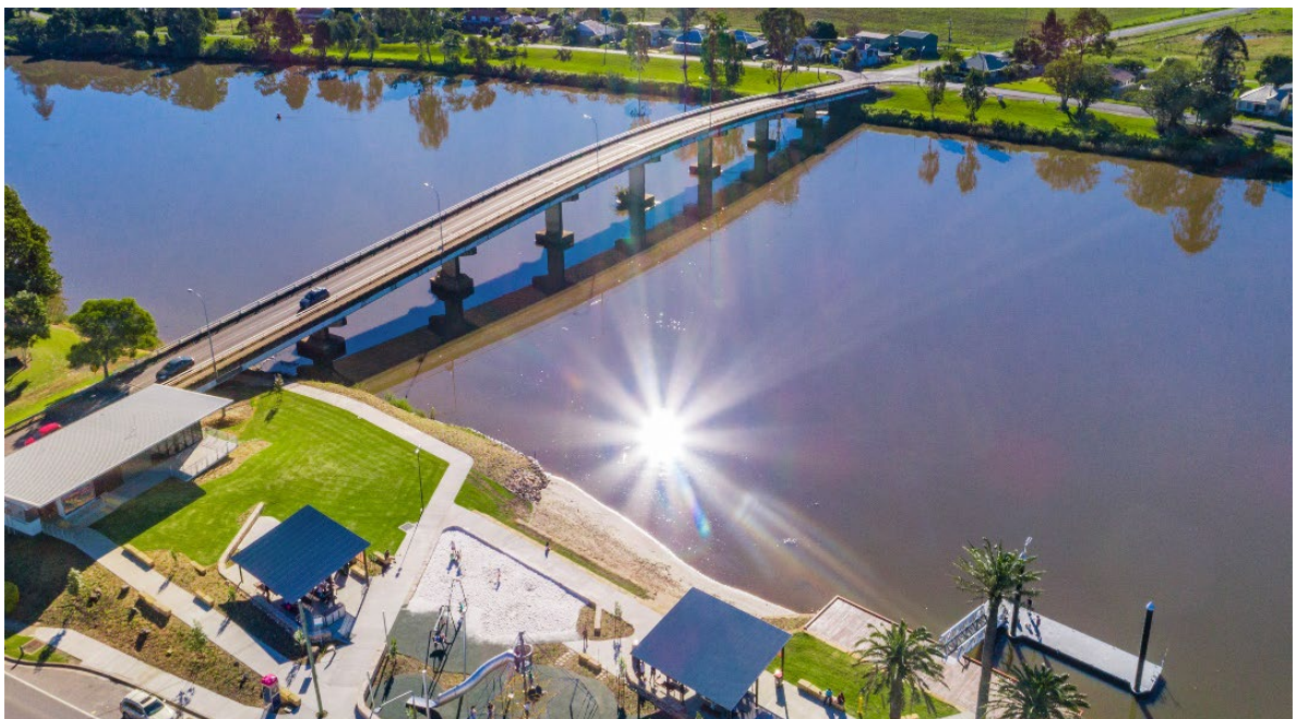
Figure 5 New pontoon located at Woodburn along the Richmond River. Photo courtesy of Richmond Valley Council.
