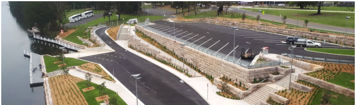
Figure 2 Boat ramp facility at Tench Reserve, Penrith, along the Nepean River.
